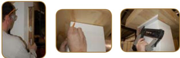
**9** Finally, attach the cap and the base to the column shaft, positioning directly up to the squaring blocks. Apply adhesive caulk to the mitered edges at the corners. Wipe off any adhesive squeeze - out with a damp cloth. Also use the adhesive to caulk the small gap between the cap/base and the column shaft. Use lightweight spackling to fill fastener holes.
