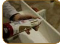
**6** With the installed external squaring blocks at the base of the column shaft, position the L-shaped sections around the support post and fasten the column shaft seams together every 6"-8" using 1 1/4" rust resistant fasteners (Important: Make sure the cleats are flush at the base before fastening the shaft together). Wipe off the excess adhesive caulk before it dries.
