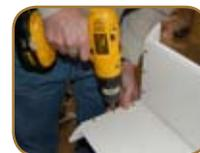
**4** If installing a balustrade railing system, pressure treated blocking must be installed at the height where the railing will be attached. Blocking is not included in the kit. The final thickness of the blocking must span the entire space between the support post and the inside surface of the column wrap. **Mounting screws must be long enough to go through the blocking into the support post for proper installation.**
